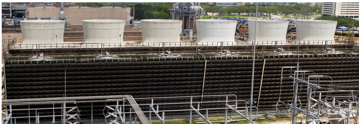
Figure 11.2 A mechanical-draft cooling tower. The fans are located within the cylindrical housings at the top. Air is drawn in through the louvers on the side.
